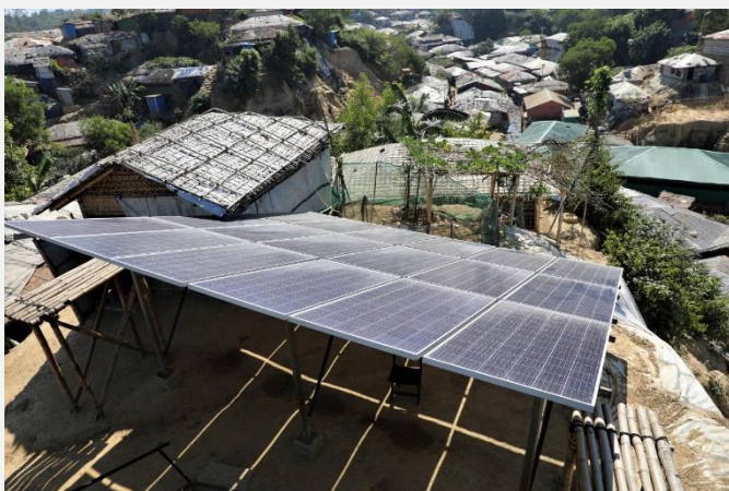
(Left) A solar powered borehole to extract ground water in Camp 11. (Right) Households in Camp 11 collect water from tap stands linked to pipelines connected to six boreholes (Photo: IFRC)
