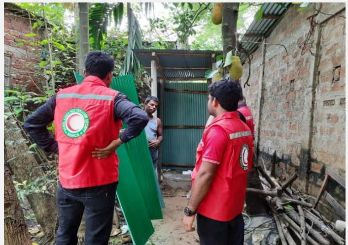
Installation of temporary latrines in Sylhet, (Photo: BDRCS)
