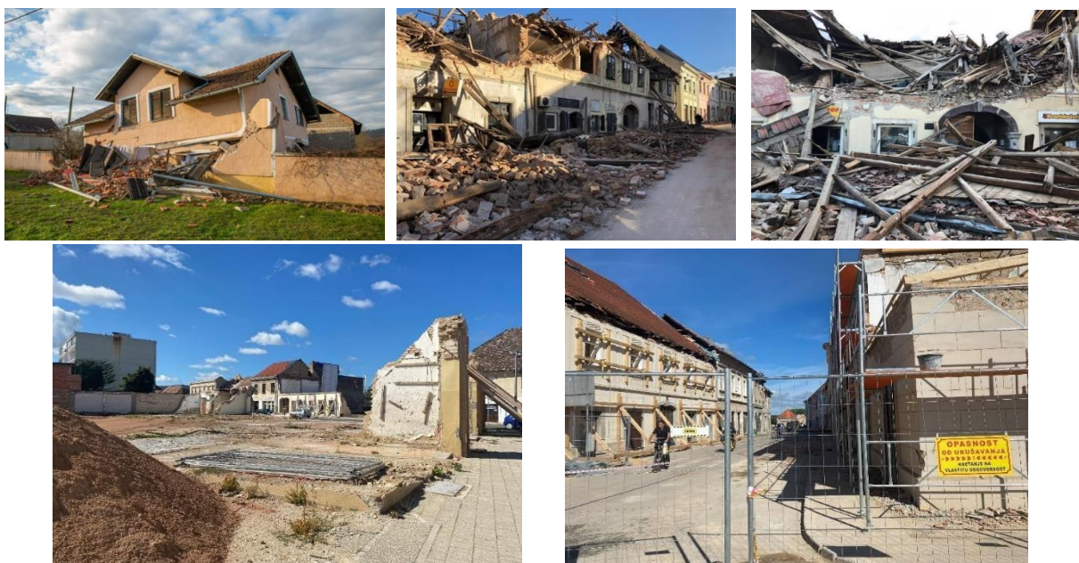
Photographs taken in the days and weeks following the earthquake on 29 December. There is still rubble and damages visible into late September as well as sites with cleaned streets from debris, removed demolished buildings and reconstruction works that started in June and July 2021. Source: CRC
