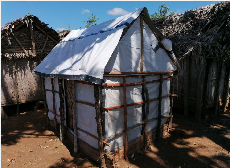
Figure 2: A temporary shelter built by the community in Sandrohy using traditional technics (Photo credit: Pascal Panoseti, IFRC)
