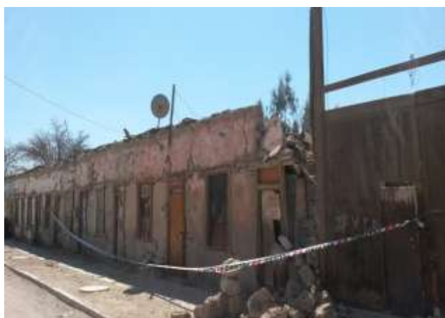
Damages to houses made of adobe in the Huara community. Source: Chilean Red Cross
