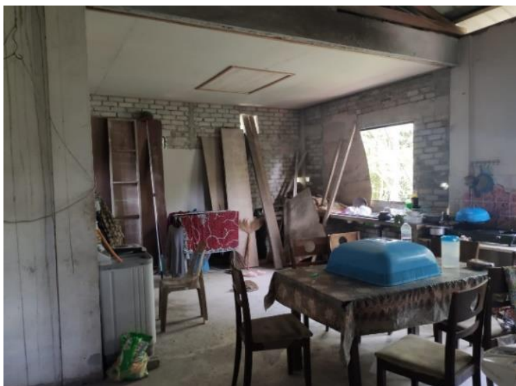
House condition of Mazlan's house in Kelantan. (Photo: MRCS)
