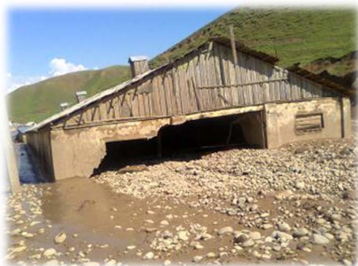
Disaster hit area. 14 April 2014. Photo: RCST
