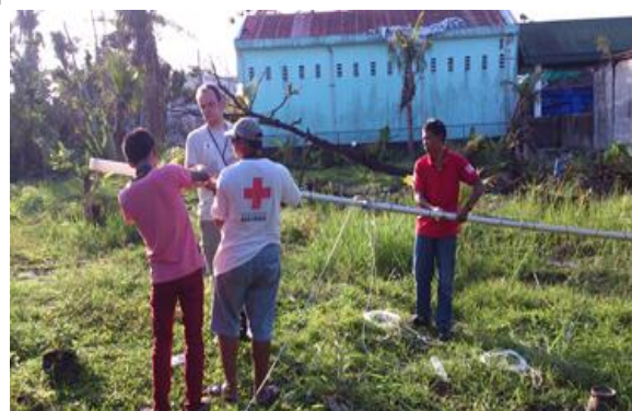
PRC volunteers carry out the installation of VHF base station for radio room operations in Tacloban. (Photo: IFRC/Charles Ranby)
