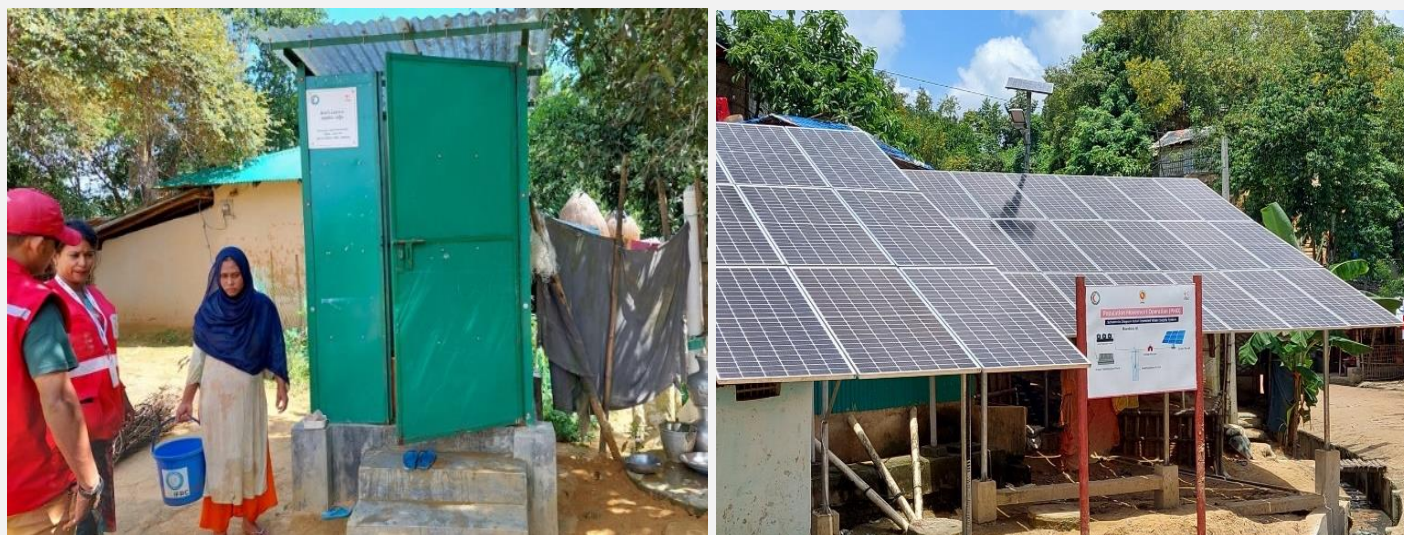
(Left) A biofil latrine in host community featured with onsite faecal waste management utilising earthworms for decomposition of faecal matter. Households using this latrine have better cleanliness and privacy. (Right) 5,500 displaced people living in Camp 19 (Block D) have access to supply of chlorinated safe drinking water from this Water Supply Network powered by solar system. Camp volunteers have been trained and mobilised to provide care and maintenance support (Photos: IFRC)
