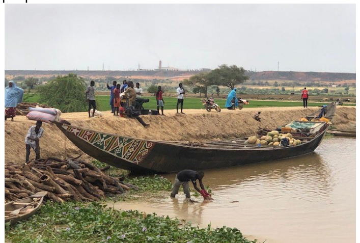
Raising the dike at Saga, Photo credit, Lamine/IFRC 8 September 2022
