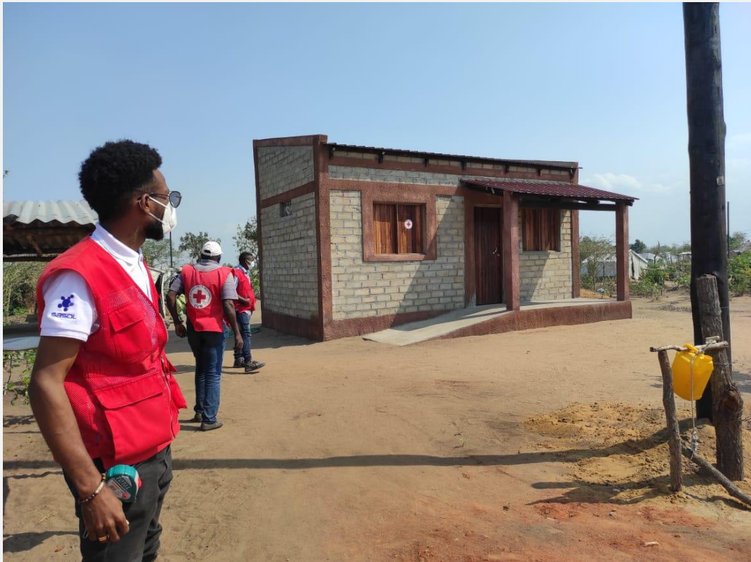
Figure 5: After- completed resilient shelter Maxiquiri 3
