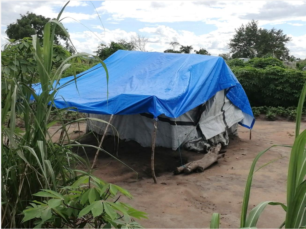
Figure 4: Before- Tarp shelter in Maxiquiri 3
