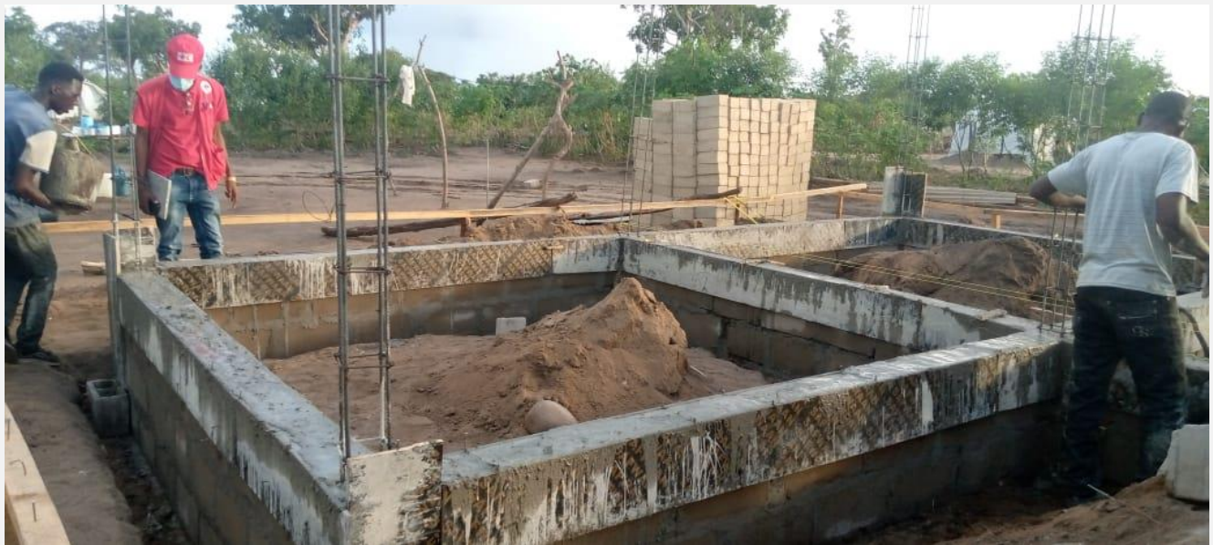
Figure 8: Practical training with master builders
