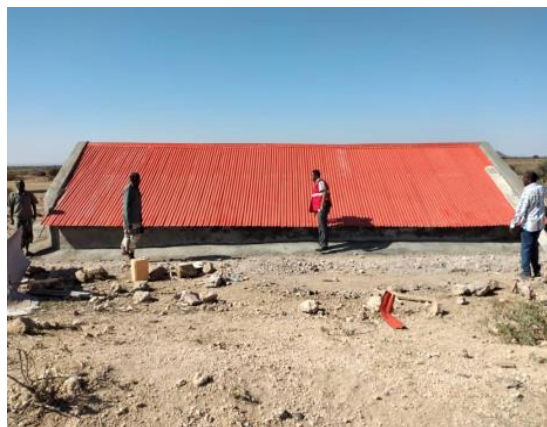
Rehabilitated berkad in Tuli Village
