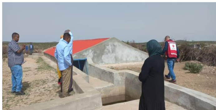
Rehabilitated berkad in Tuli village
