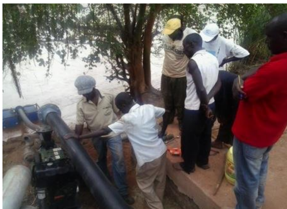
A rehabilitated irrigation pump machine in Mwingi. Photo/KRCS.
