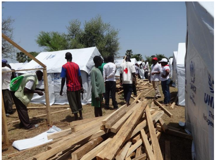
Shelter construction in Dougi by Red Cross volunteers Photo/IFRC
