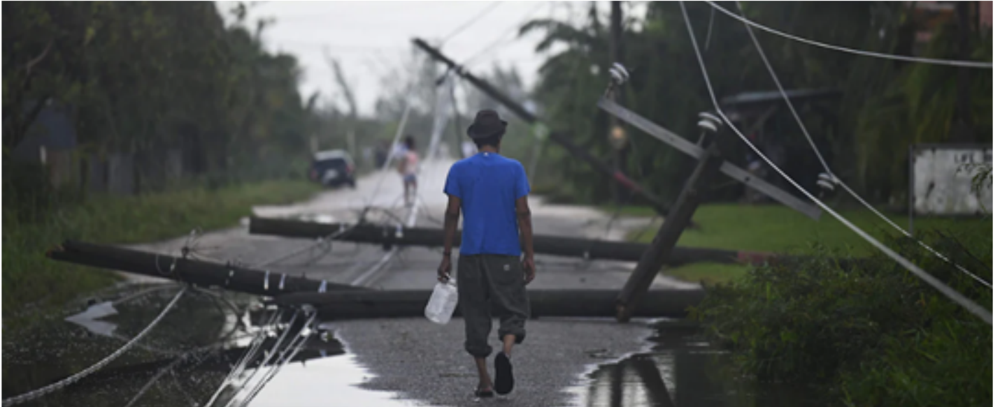
Fallen utility poles block a street in Ladyville, Belize, after the passage of Tropical Storm Lisa. Source: The Washington Post.
