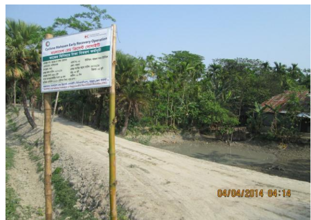
Road repaired through cash for work. Photo: IFRC
