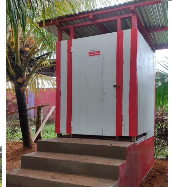
Construction of community latrine RACCN, December 2021. Source: NRC.
