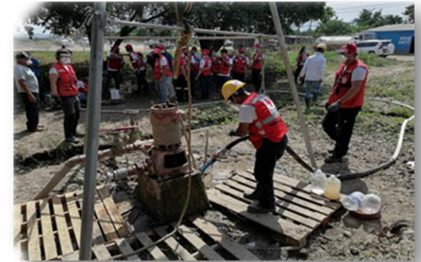
Well cleaning in the community of Guaruma 1, March 2022. Source: HRC
