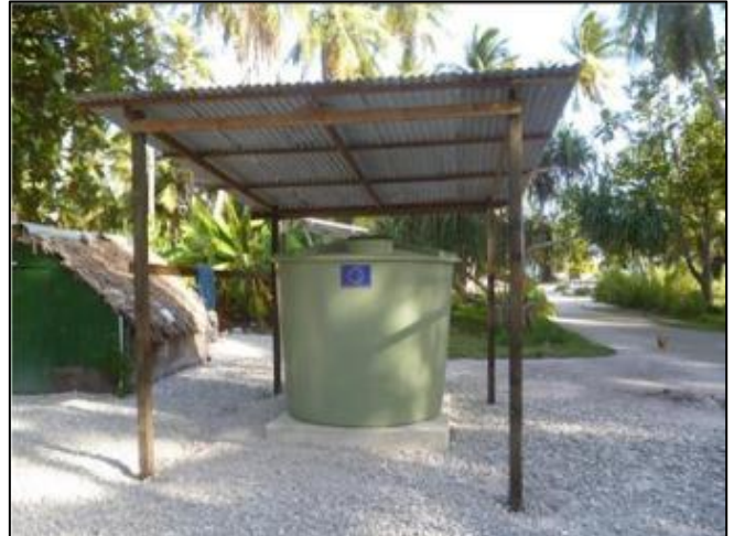
An example of a new catchment structure which was installed where existing roofs were inappropriate for rain water harvesting. The rainwater tank was supplied and installed by IFRC on Majkin Island, Namu Atoll in January 2014. Credit: Ana Zarkovic/IFRC
