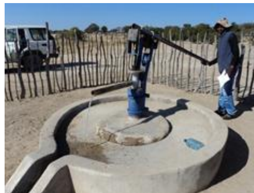
Sikwakweni borehole ward 3 rehabilitated. Photo: IFRC
