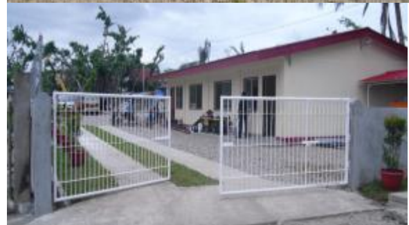
Before and after the storm: The chapter office building itself mostly survived the onslaught of Haiyan, though its compound had to be completely rehabilitated. A donated prefabricated structure also provides essential office space in the resurfaced compound area. (Photos: PRC/IFRC)
