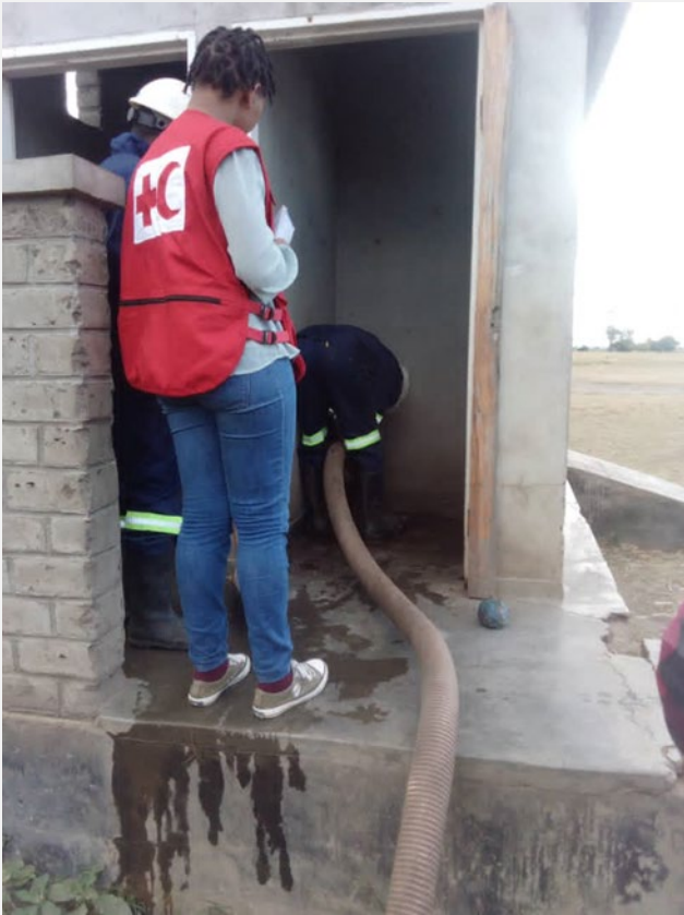
• Desludging a pit latrine at a school in Chikwawa District @MRCS
