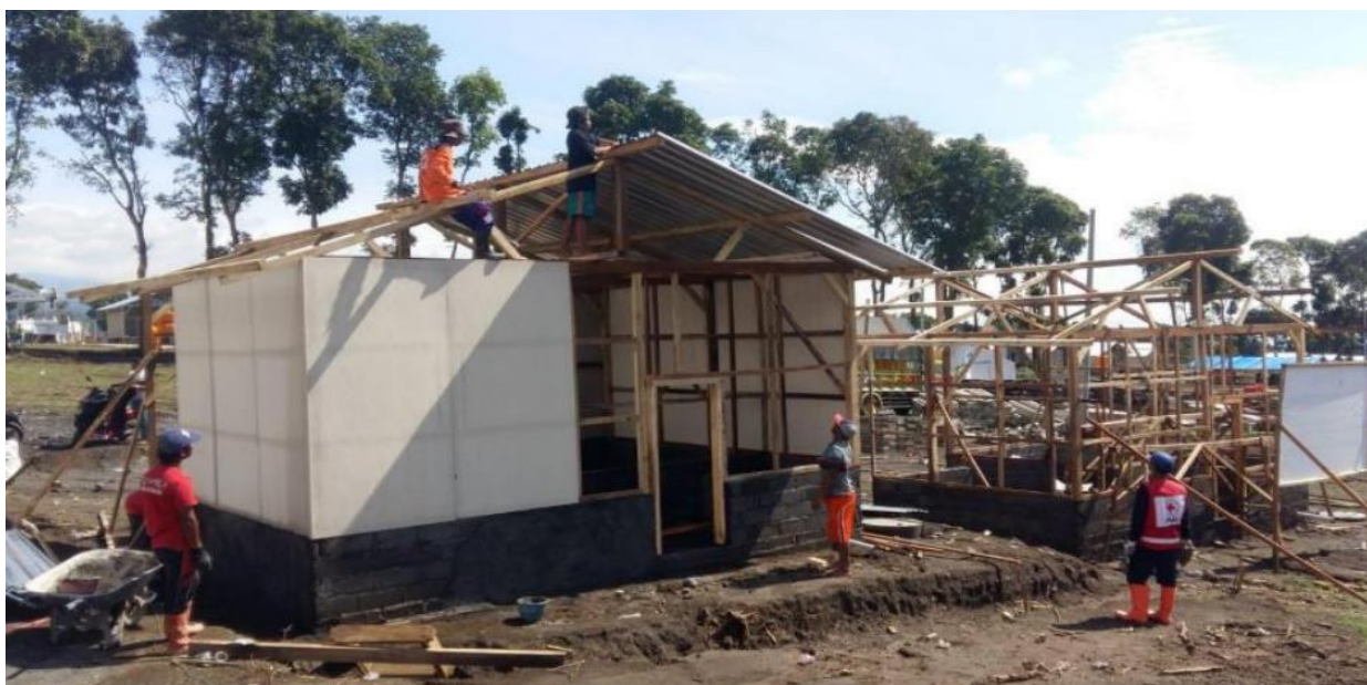
Construction of a temporary shelter in progress. (Photo: PMI East Java)
