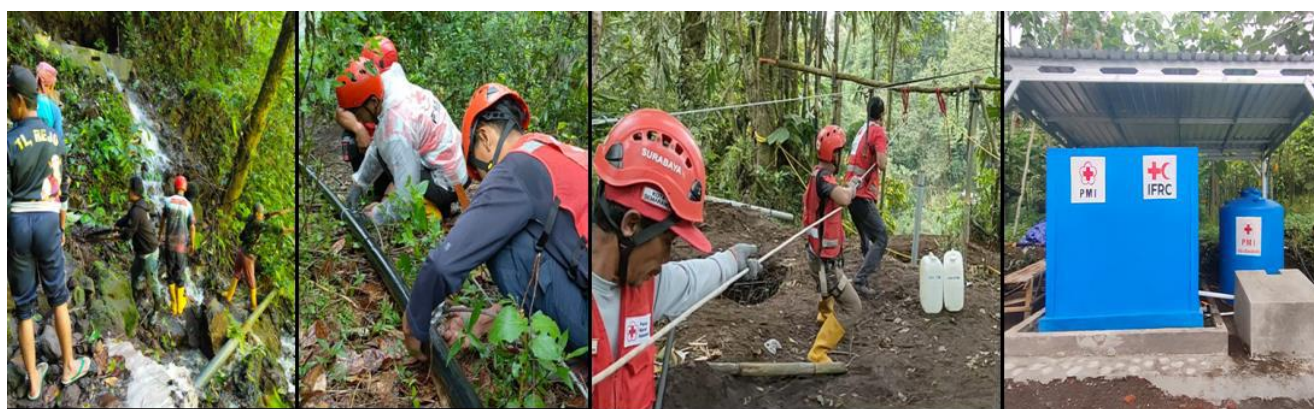
Pipeline construction process. (Photo: PMI East Java)
