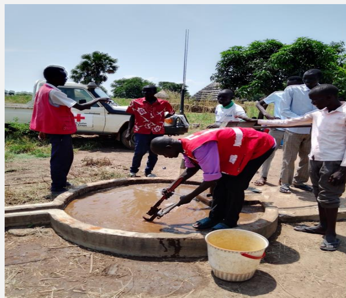
Pumping water after successful rehabilitation in Aweil South.
