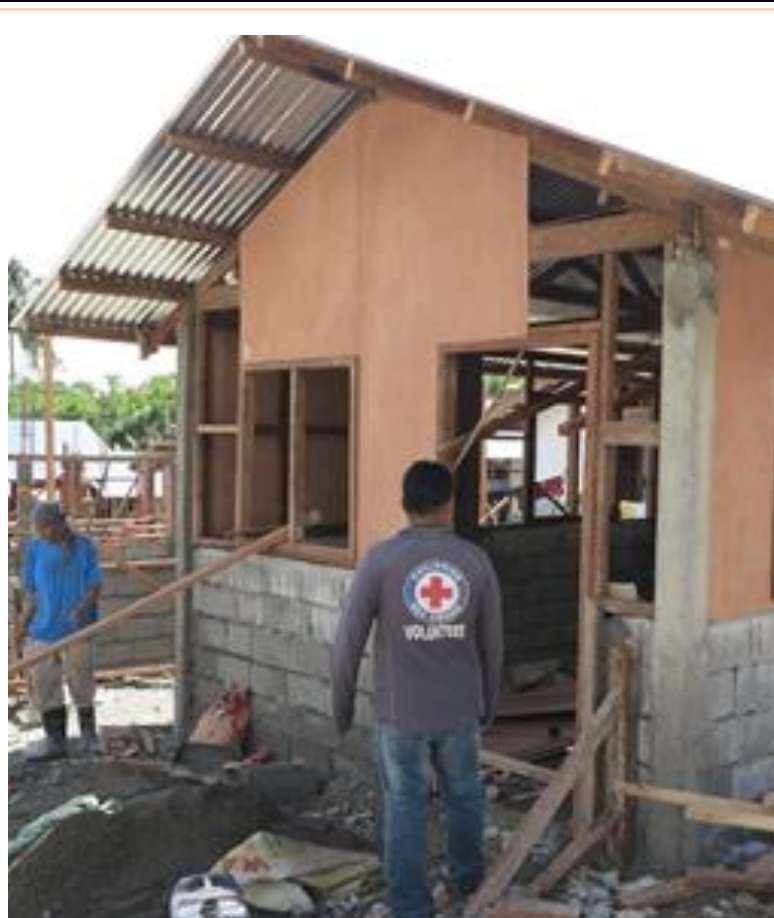
A Red Cross volunteer monitors the construction of transitional wooden and concrete shelters in a relocation site in the province of Davao Oriental.
