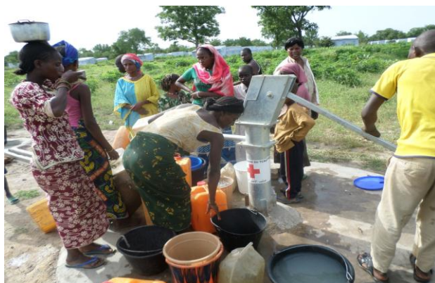
A total of 10 water points were constructed in the area of intervention, providing returnees with access to safe water. Photo/RCC.
