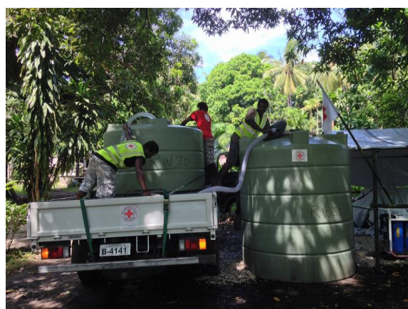
Water from a borehole in Tertere Correction Facility is treated with a NOMAD water purification unit and delivered to communities in Guadalcanal plains, 2014. Photo: Ana Zarkovic / IFRC.
