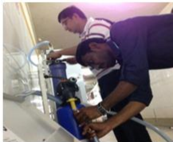
Installation of WPU in Bone and Joints Hospital Srinagar.
