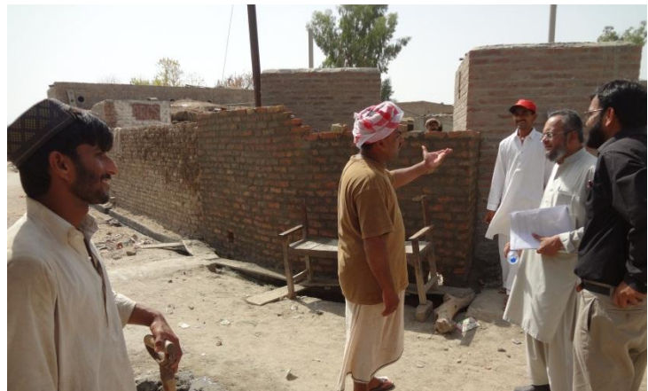
A Beneficiary constructing his boundary wall
