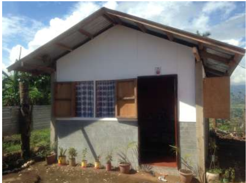
A Red Cross typhoon-resilient shelter built with concrete and wooden materials. A total of 800 of this type were built in Bopha affected areas.
