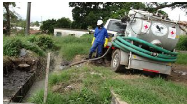
Desludging of latrines in Blantyre. Photo: MRCS
