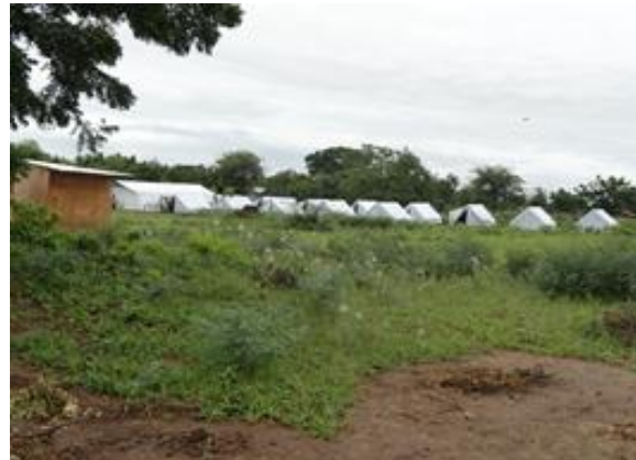
Emergency Shelter constructed in Magoti camp. Photo: MRCS
