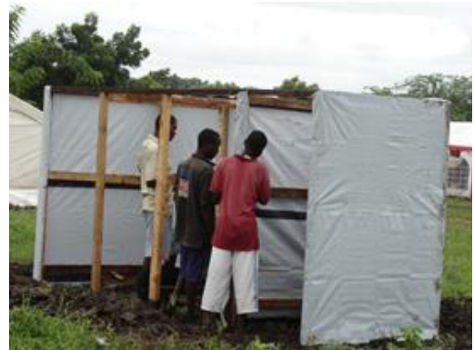
Latrine construction in Magoti camp. Photo: MRCS
