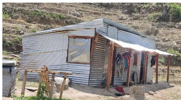
Figure 21: A transitional shelter constructed under this assistance using CGI sheets all sides covered
