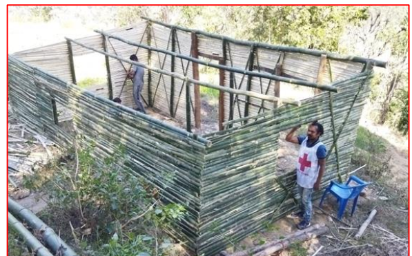
Figure 20: A transitional shelter being constructed at the beneficiary's premise. (Source: NRCS)
