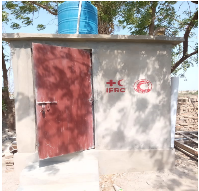
Latrine constructed by PRCS in Larkana, Sindh (Photo: Review team)
