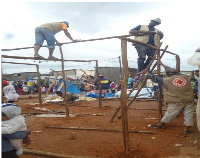
CRM volunteers support the construction of temporary shelters © CRM
