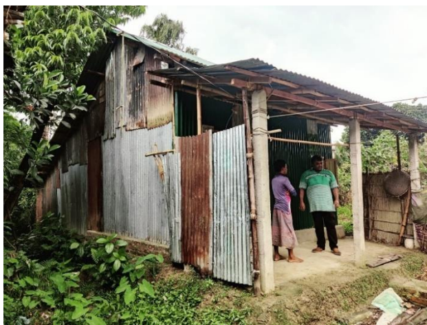
Photograph 2: Some of the most disadvantaged households could not afford to contribute for the wall materials. They used straw, bamboo or their old CGI sheets as wall materials
