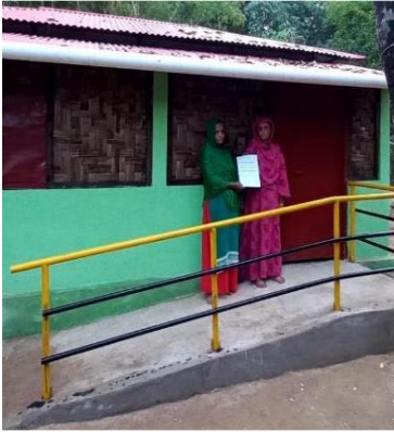
Figure 5. Modified shelter with a ramp and railing to enable a person with disabilities to access the house. (Photo by BDRCS/American Red Cross)
