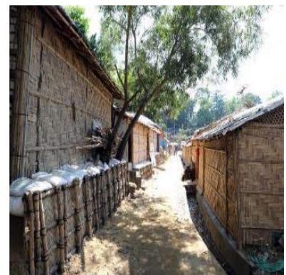
Figure 6. A mid-term shelter in Camp 12 with a guide wall to protection from flood or rainwater in the monsoon. Photo by BDRCS
