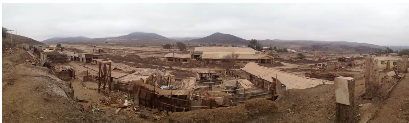
Several houses in the town of El Salado have been completely destroyed. Source: IFRC
