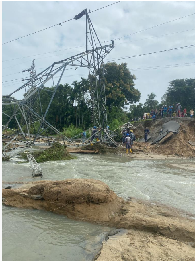
The major road and electrical supplies from the electricity plant in the Ampara district were destroyed by a flash flood resulting from extreme weather conditions. (Photo: SLRCS)
