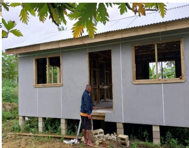
Figure 9. MoI house under construction in Fonoi. Photo: TRCS
