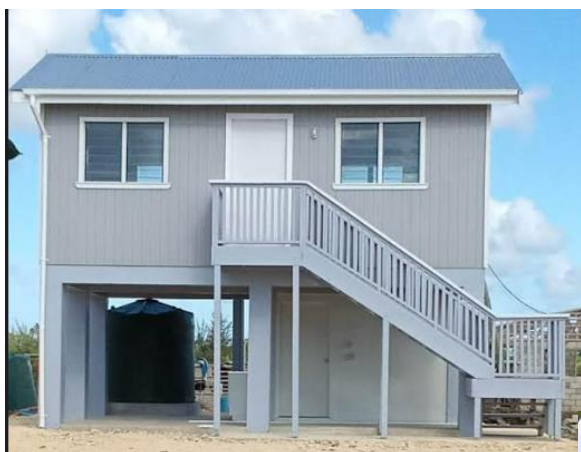
Figure 8. MoI house built in Tonganapu. Photo: TRCS
