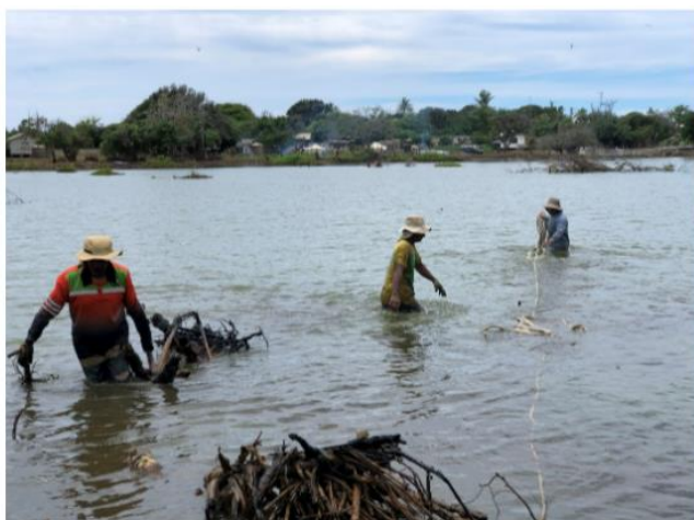
Figure 10. Ropes were used to tie debris together. Photo: TRCS
