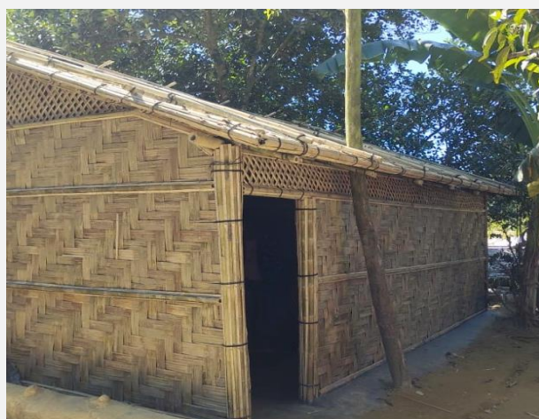
(Left) A Completed mid-term shelter made of bamboo in Camp 4. (Right) A durable shelter was constructed for one of the vulnerable households in Teknaf host community. (Photo: IFRC)
