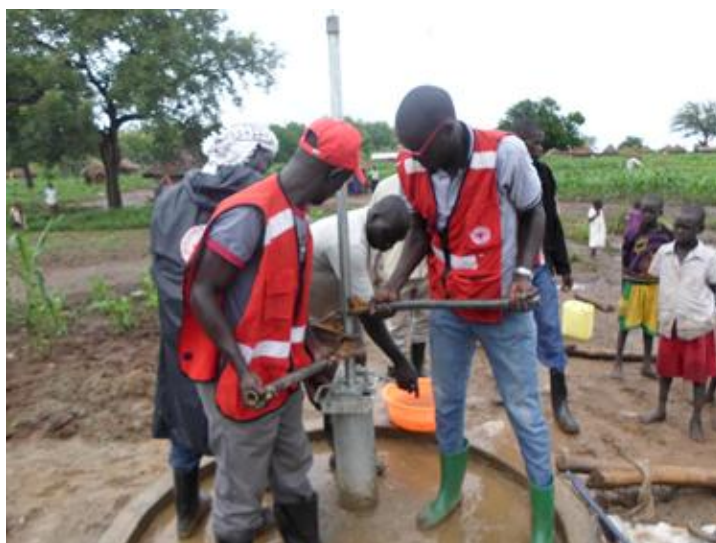
New borehole drilled and equipped. Photo: URCS
