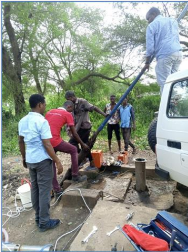
Borehole rehabilitation in Bondeni, Tana River County. Flushing, disinfection and replacement of pump parts. (KRCS Photo).
