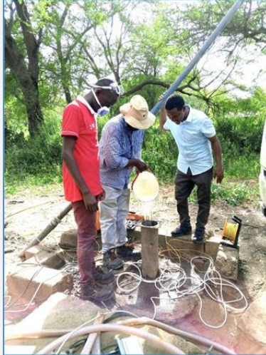
Borehole rehabilitation in Bondeni, Tana River County. Flushing, disinfection and replacement of pump parts. (KRCS Photo).
