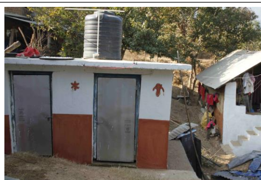
Support for latrine construction
