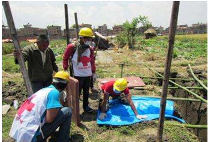
Nepal Red Cross Society team constructing temporary toilets at one of the camp sites. Photo: NRCS.
