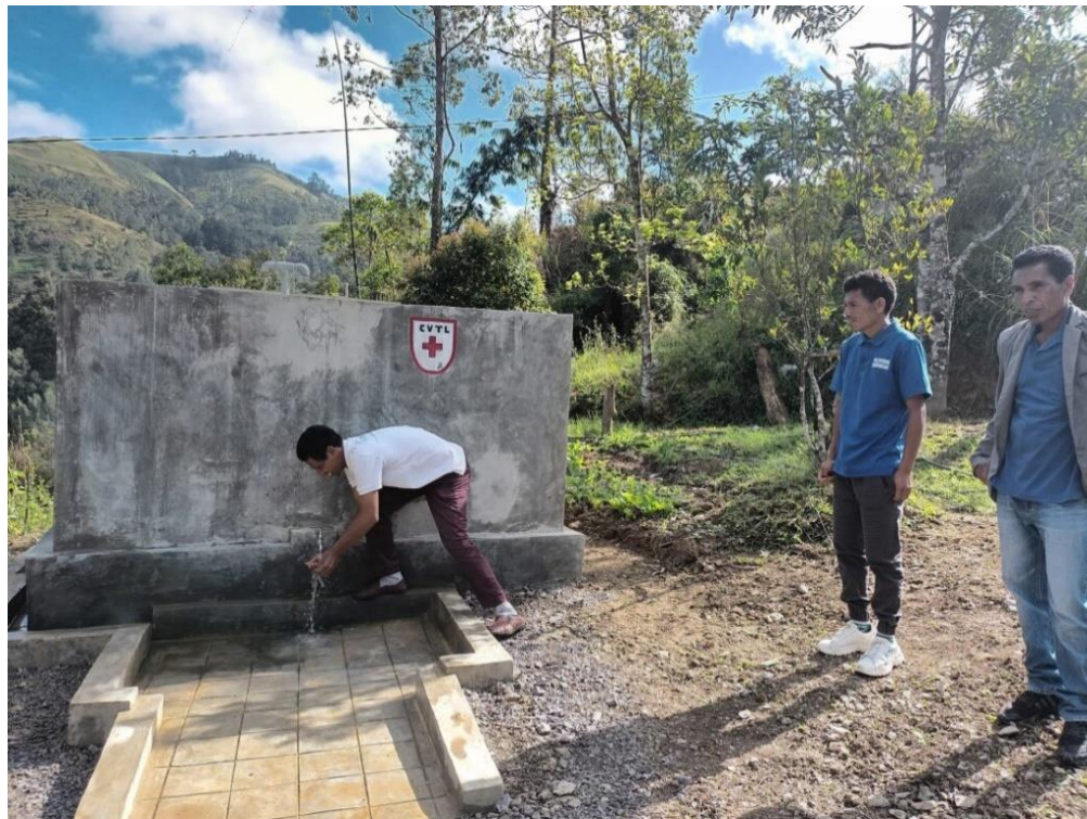
Photo 10. Water Facility in Manelobas
