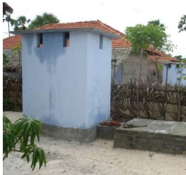
Well completed latrine
