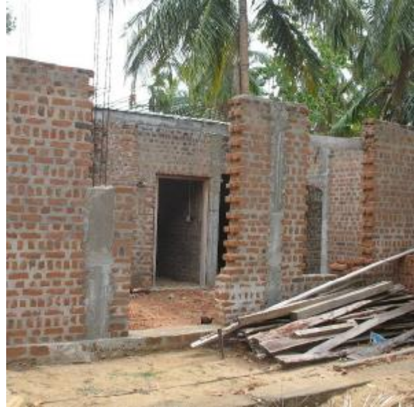
Incomplete house in Pottuvil
