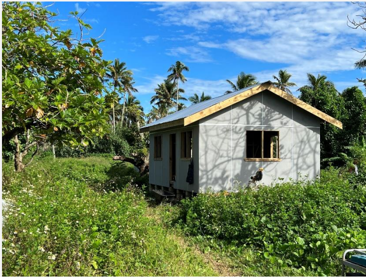
Tsunami House still on progress. (Photo Credit © TRCS 2023)
