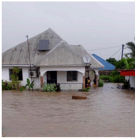
Flooded house in affected community
