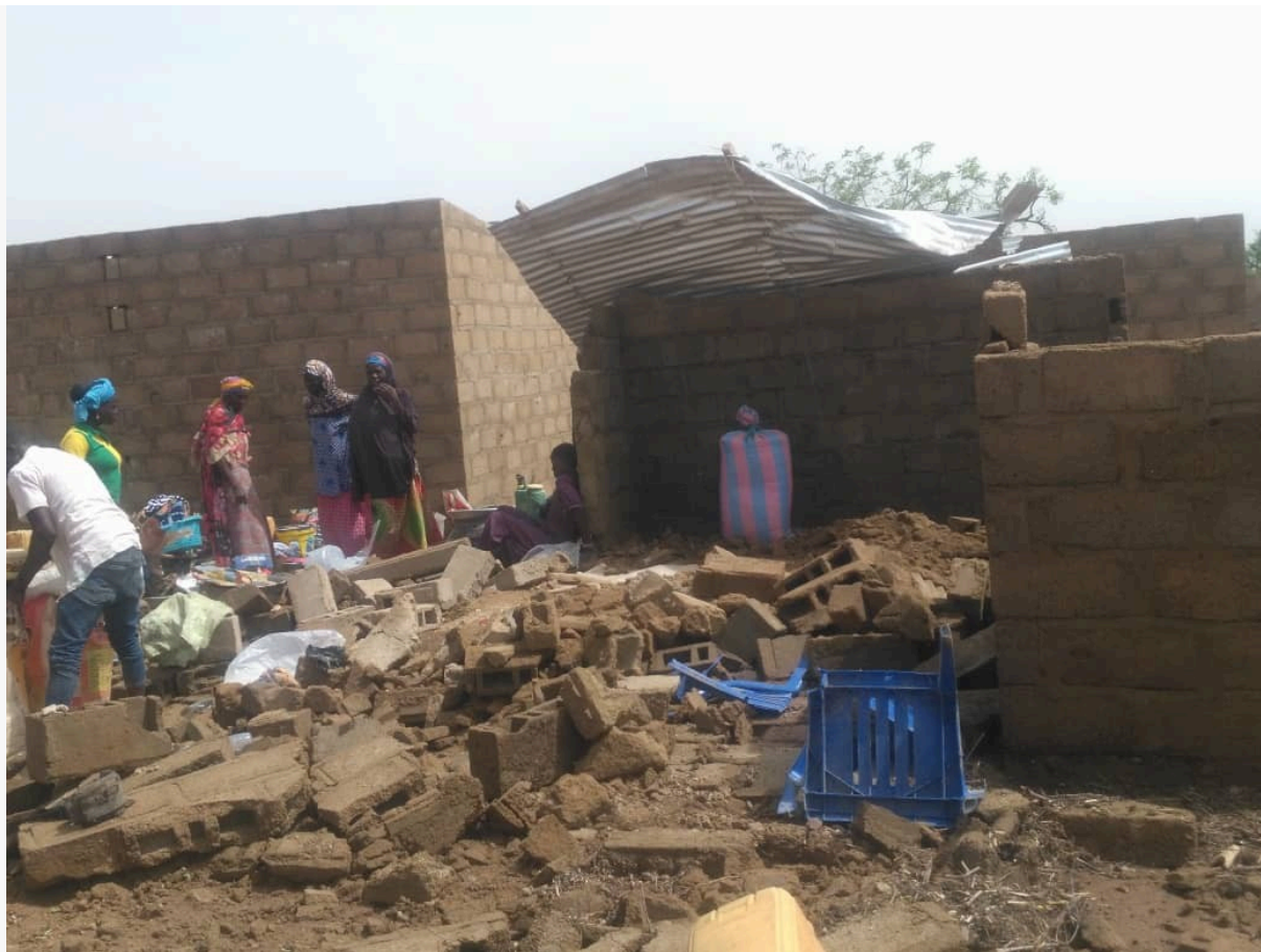
Collapsed houses in Boulsa
