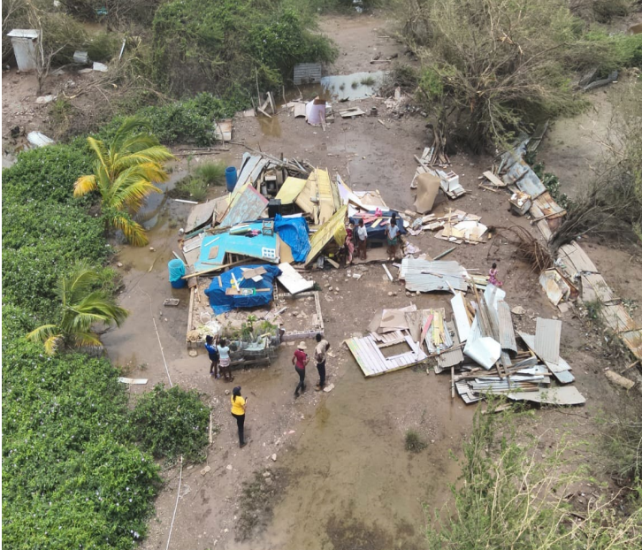
Homes and structures destroyed by Hurricane Beryl in Clarendon, Jamaica (ODPEM).
