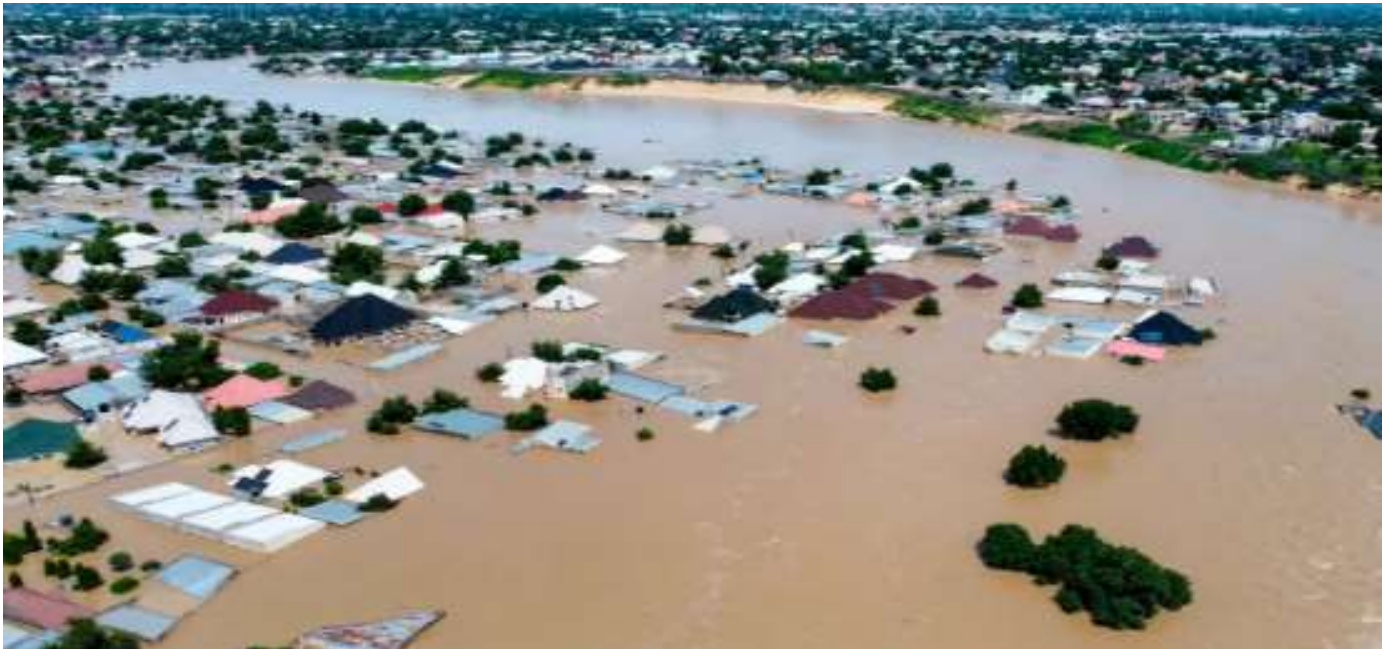
Submerged buildings in Maiduguri, Nigeria on 10 September 2024. (Photo credit: Musa Ajit Borno/AP Photos)
